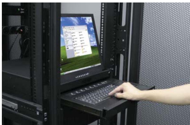
Figure 7. Operating the LCD keyboard drawer.
